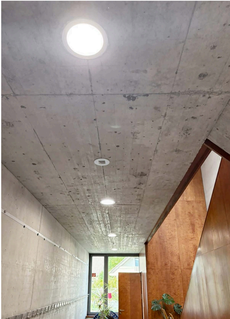
Downlights MARS | ©AKA Leuchten AG
